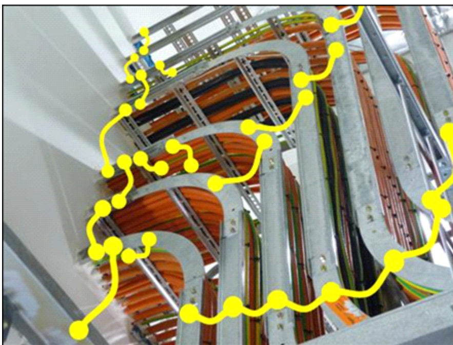
Figure 8-7 Examples of bonding natural metalwork, on an existing synchrotron, #3.
