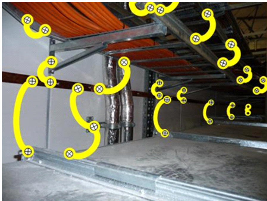
Figure 8-6 Examples of bonding natural metalwork, on an existing synchrotron, #2.
